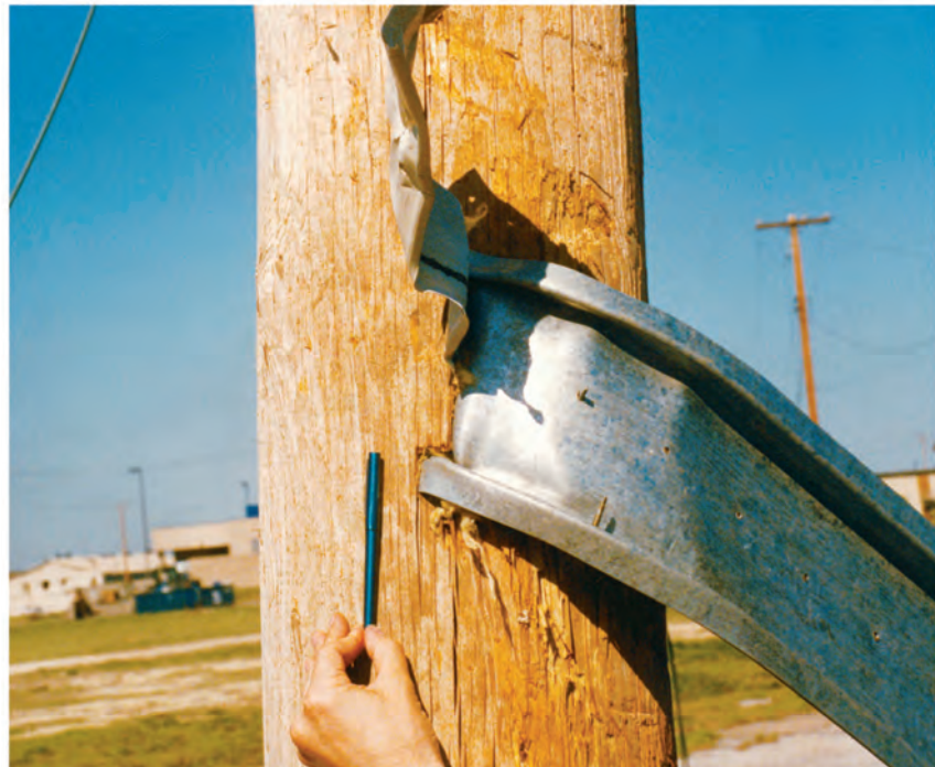
FIGURE 1 Tornado Damage The force of the wind during a tornado was strong enough to drive a piece of metal into this utility pole.
