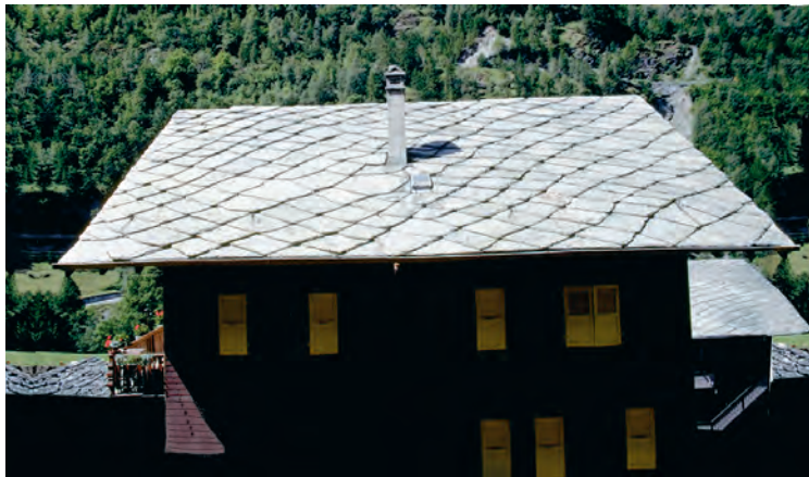
FIGURE 4 Slate The roof on this house is made of slate. Slate is a metamorphic rock that forms from the sedimentary rock shale.
