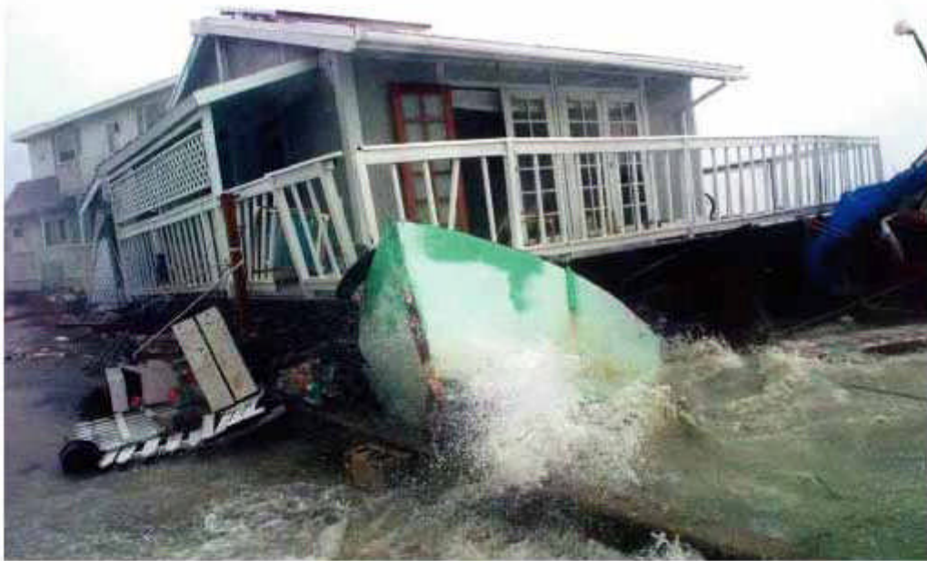
Figure 9 A hurricane's storm surge can cause severe damage to homes near the shoreline.
