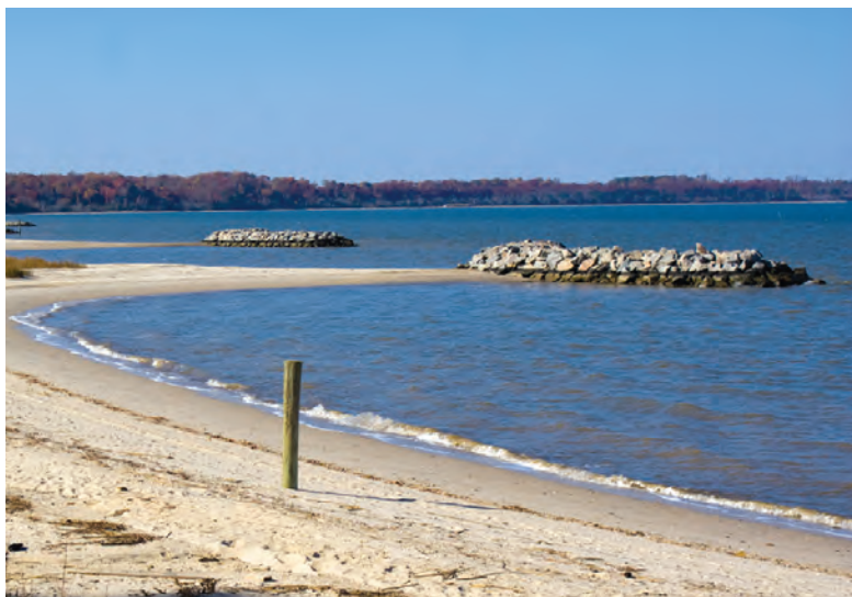
FIGURE 24 Breakwater These breakwaters, built along a Chesapeake Bay shoreline, should help protect the shoreline from erosion by absorbing force from strong waves.
